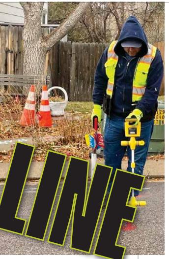
White lining demonstrates a respectful approach by clearly indicating the confines of the excavation area. This action prevents accidental encroachment onto neighboring properties, minimizing disruptions, and upholding the boundaries of shared spaces. It showcases an understanding of the importance of respecting the properties and spaces of others, fostering positive relationships within the community.
