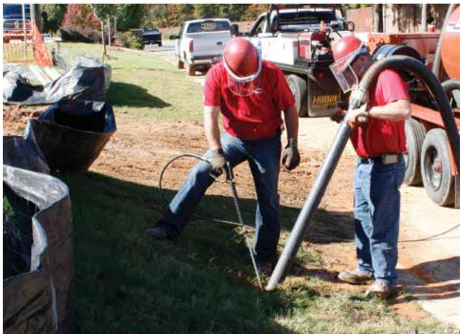
24” on either side of the utility, though some states go as wide as 36”. Within this area, mechanical excavation is restricted, and hand digging or approved soft-digging methods are required.
