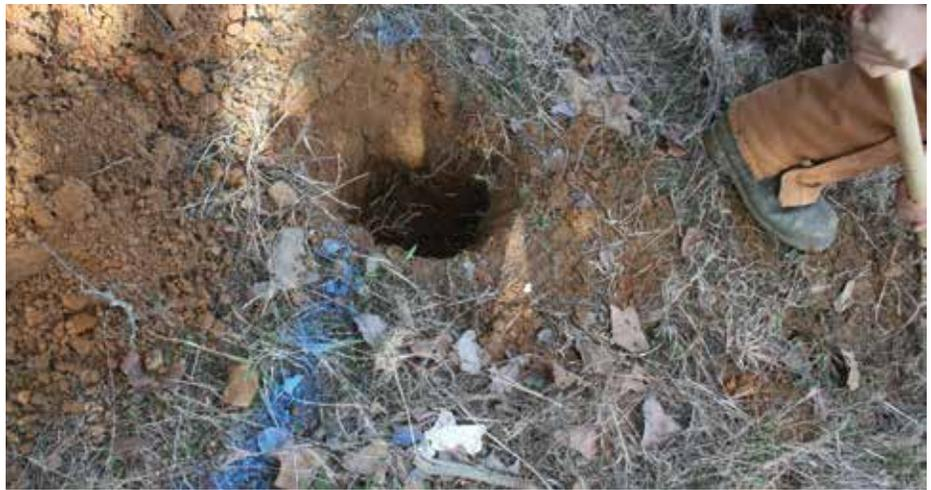
often have multiple utilities stacked in the right-of-way. Mechanized equipment is risky in these conditions. Hand digging allows the precision needed to separate and identify each facility safely.
